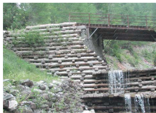
Figure 1.20 - Check on compensation works
