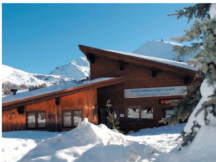
Figure 2.17 - Weather Local Centre, Sestriere
