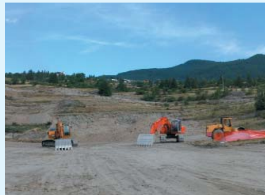
Figure 1.11 - First excavations at the site for the Freestyle run
