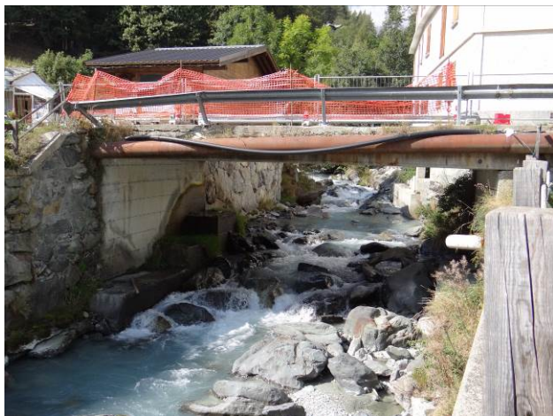
Ponte strada Balme-Fraz. Cornetti
