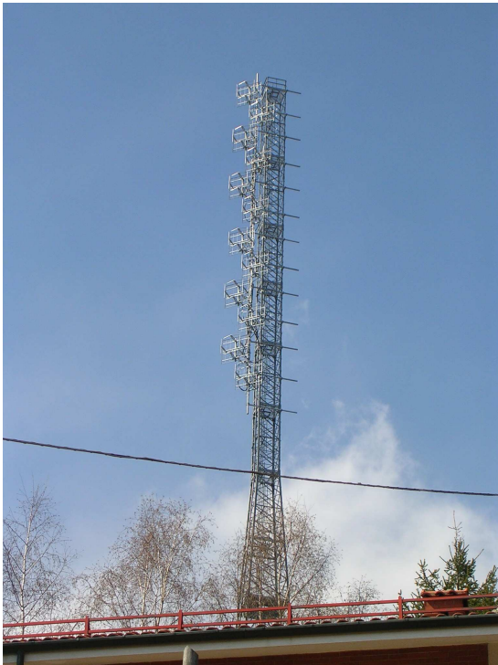
Plant A ( f=102.5\text{MHz} ): H=30\text{m}
